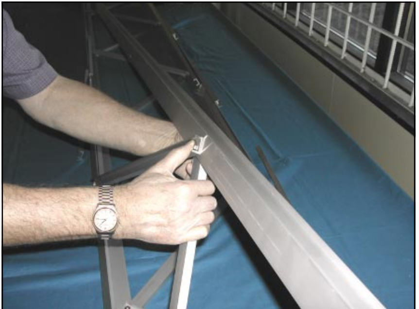
The very first connection to be done to the third corner leg. Here a three material holding a screw M6x20 along with washers and nut
