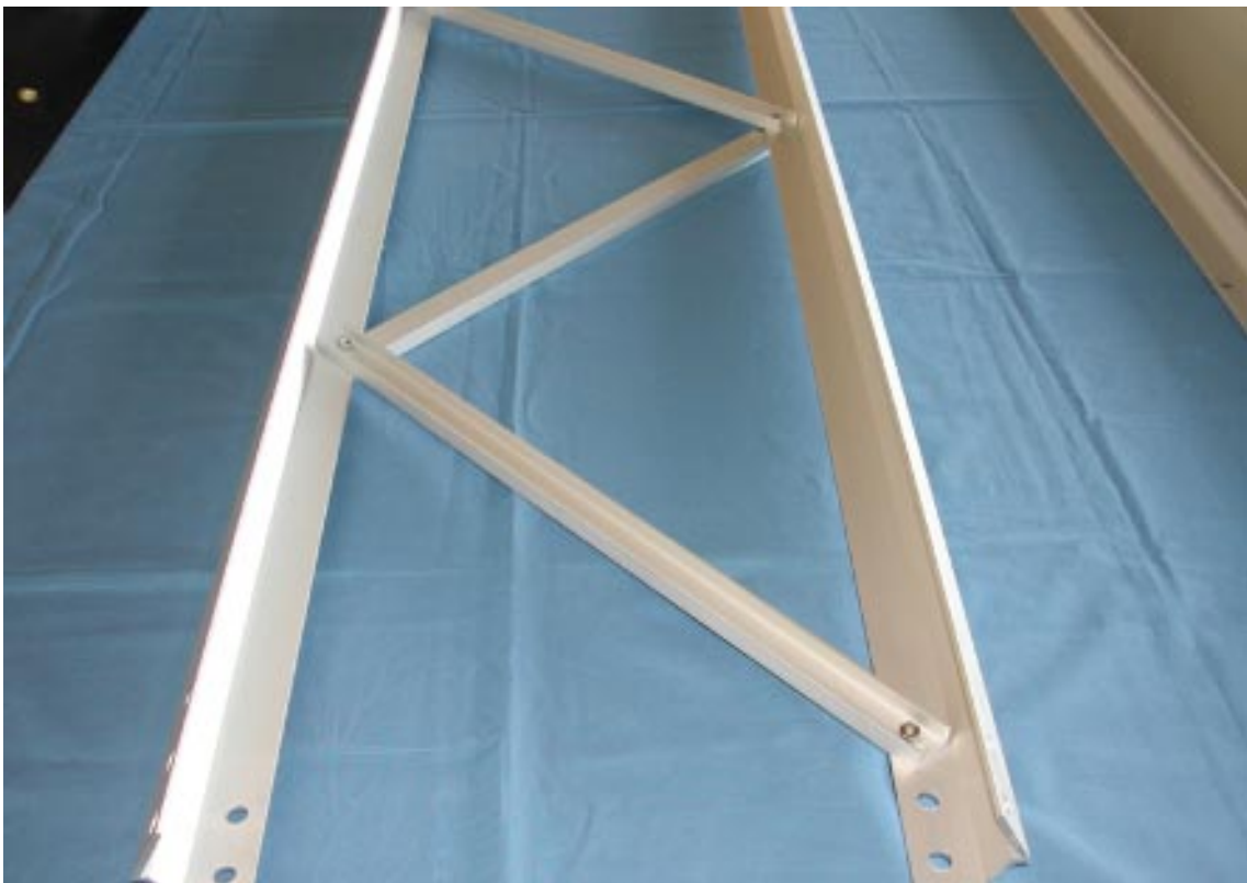
The beginning of a middle section having strays mounted without having the bolts tightened.
